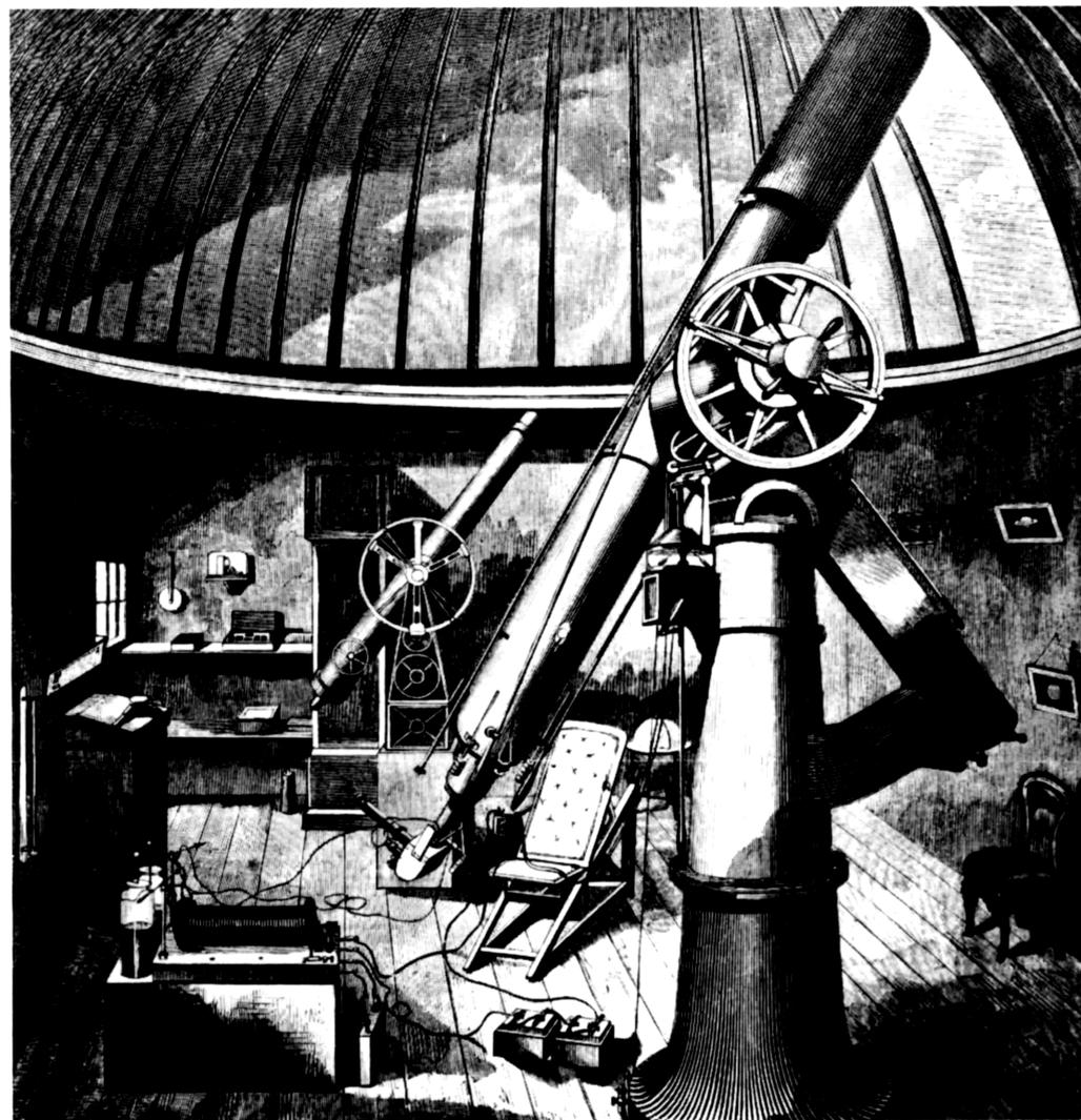
The Huggins observatory at Upper Tulse Hill, near London, had a 12-foot dome. The 5-inch Dollond refractor occupies the transit room, in the background here, and the 8-inch Clark-Cooke refractor is mounted in the main dome. This is what the interior of the Huggins observatory looked like between 1860 and 1869. Later, larger instruments were installed. Pictures of planets hang from the wall. (from *An Atlas of Representative Stellar Spectra*, 1899)
